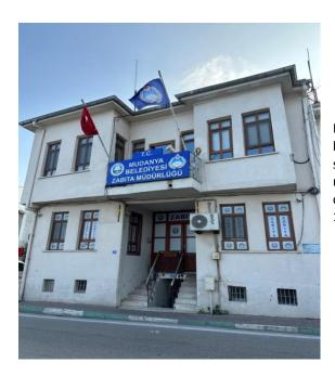
The building, located on Mustafa Kemal Paşa Avenue in Mudanya Şükrüçavuş Neighbourhood, was constructed as a 2-storey building atop the basement. The windows on the basement floor are small square, while the windows on the other floors are vertical rectangular. The floor covers, ladders and roof of the building are made of wood. The building, which had been used as Mudanya City Hall until 1976, is now used as Mudanya Municipal Police Department.
