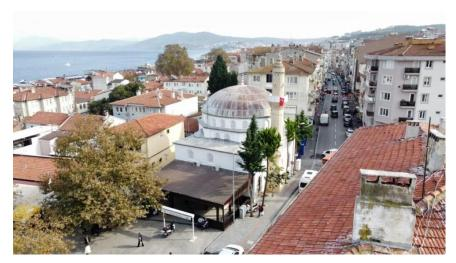
Located in Mudanya downtown, the mosque was renovated with a large-scale repair in 1975 and only the minaret is in its original condition. The minaret, made of ashlar, was damaged in the earthquake in 1999 and the top of the minaret balcony was renovated. The flat roof of the square-planned mosque, which was repaired in 1975, has been covered with a dome.
