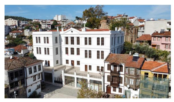
In the building constructed in a neo-classical style, natural building materials were used in accordance with the construction system of the period. Although baked bricks are the main materials of the masonry system, solid stones were also used in the direction of the slope in the external wall masonry. The interior and exterior walls were plastered, and the exterior wall decorations and surface of brick columns were made of hard plaster with additives.
