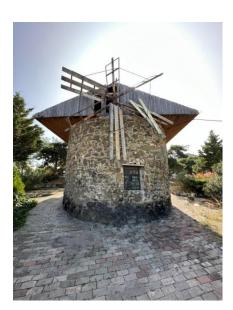
The height of the mill, which was modelled after the windmills previously operated in Mudanya, is 4.60 m and the cylinder diameter is 5.20 m. The walls of the building were masoned with rubble and crushed stone mortar. Its six-bladed propeller, made of iron and wood, was designed to rotate with the wind. It had been used as a flour mill for many years and as an ammunition store during the war years. Today it is located above the park.
